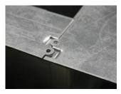
If it is jointed, you can not disassemble without tools such as a flathead screwdriver.
